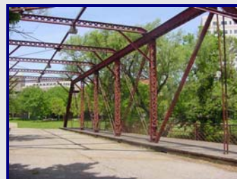
Client: City of Trenton Location: Trenton, NJ Services: Construction Inspection
