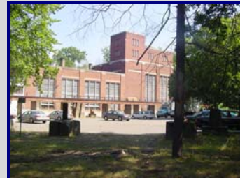
Client: NJDPMC Location: Trenton, NJ Services: Survey & Civil Engineering
