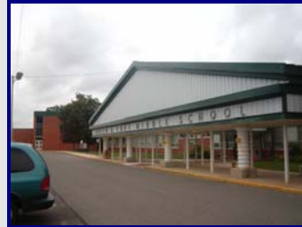
Client: NJSCC Location: Pemberton, NJ Services: Construction Management
