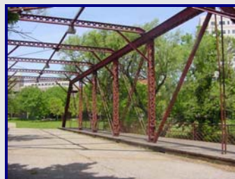
Client: City of Trenton Location: Trenton, NJ Services: Construction Inspection
